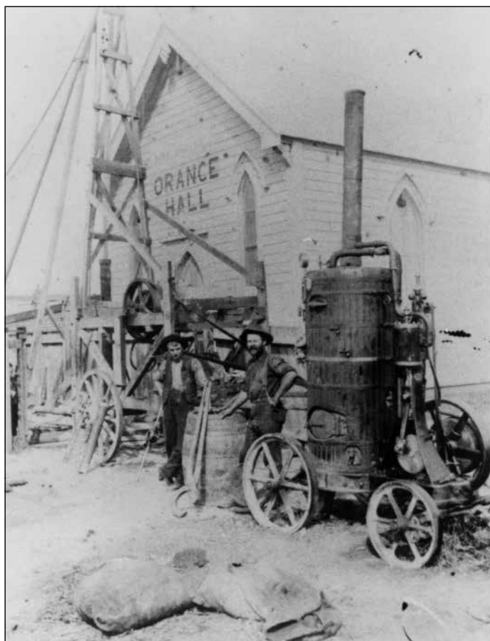
Figure 1.9: Well drilling at Hastings in the early part of the century. Alfred Ferdinand Leipst (on right) drilling a well outside the Orange Lodge Hall, Warren Street, Hastings. (photo: print donated by George Willan, Hastings).
