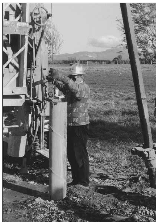
Figure 1.15: Dick Baylis checking progress during drilling of the HBRC Flaxmere testbore (well no. 3698 3 ) (photo: Len Brown, IGNS).
