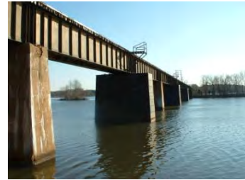
LAKE GASTON BRIDGE
