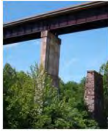
TAR RIVER BRIDGE
