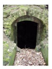
A huge circular structure part set into the ground, 30ft diameter and 25ft from floor to ceiling. Built of stone with a magnificent domed brick roof and insulated by a layer of soil. It is a 10ft drop from the door to bottom which would be filled with ice from the ponds.
