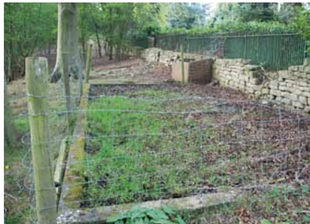
5. View of dry stone wall and iron railing detail forming a boundary to the perimeter estate footpath. An existing water collection point exists adjacent this.
