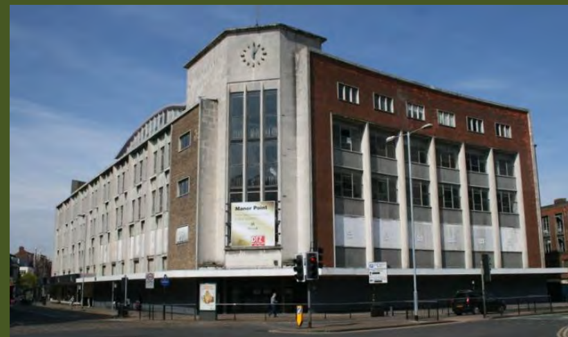
Former Co-operative Department Store. Bond St-Jameson St, 1959-61
