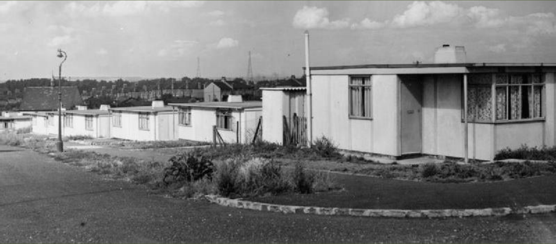
Prefabs on housing site in Hull cleared after bomb damage
