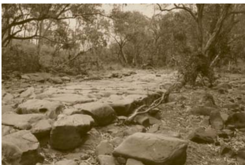
Causeway on the Bump Road, Hodgkinson goldfield
