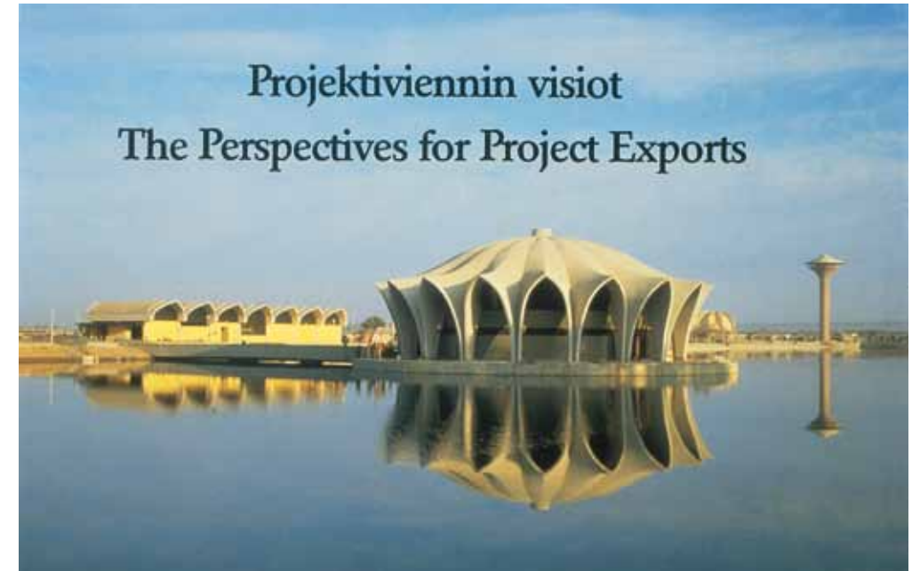
Yleinen Insinööritoimisto erected a beautiful recreation centre in Baghdad, Iraq. The centre was intended for the Conference of the Non-Aligned Countries. The project was completed in 1982, during the peak era for Finnish construction exports. This photo is taken from a brochure for an export seminar held in Helsinki in 1987. However, the good years for construction exports were over, in spite of hopes to the contrary.
