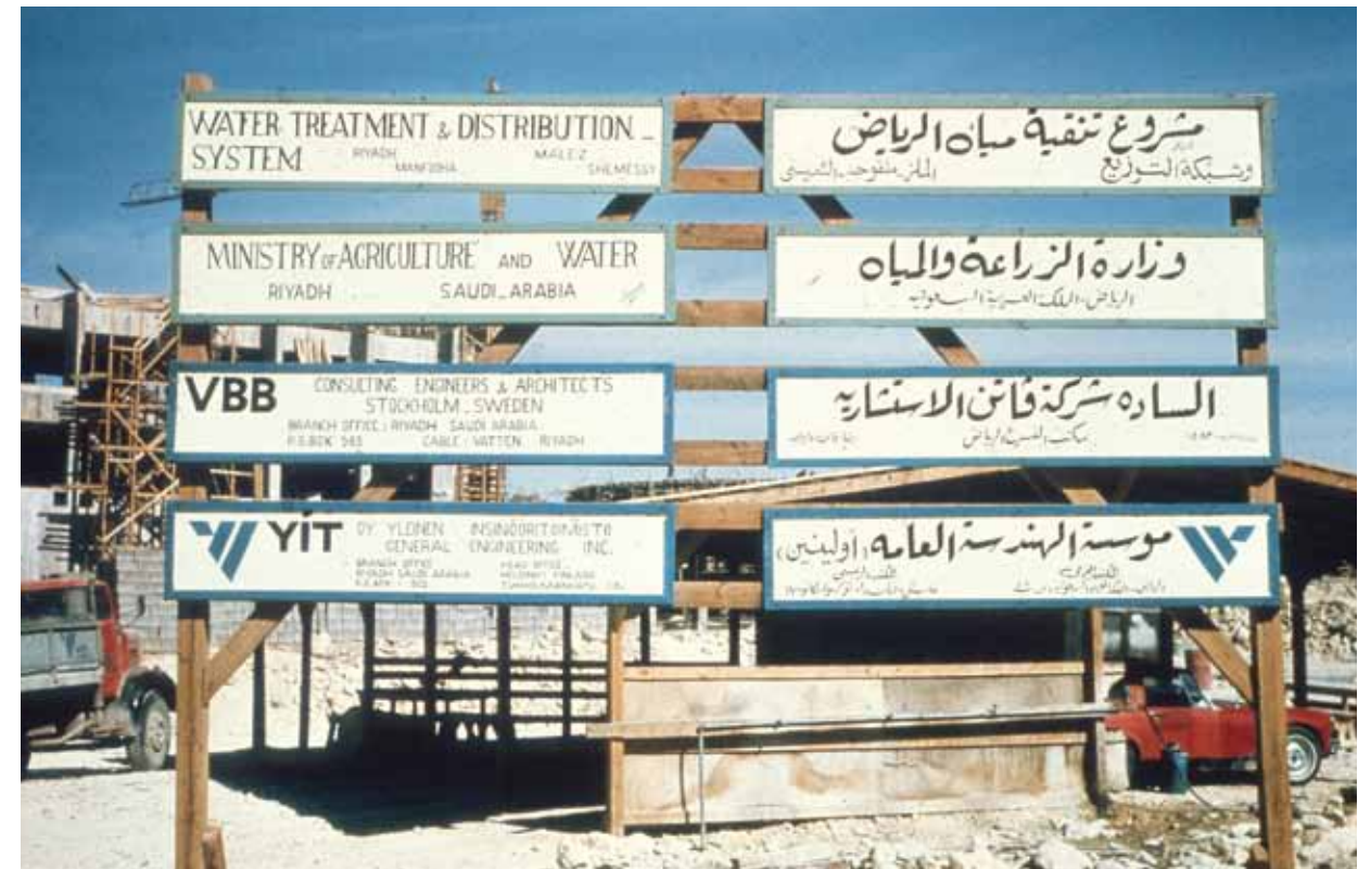
Waterworks construction site signs in Riyadh, Saudi Arabia. Yleinen Insinööritoimisto (YIT) built the facility from 1967 to 1972.
