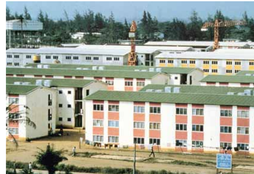
Perusyhtymä Nigeria Ltd built a high-rise community for army personnel in Lagos, the capital of Nigeria, in 1977–1979.
