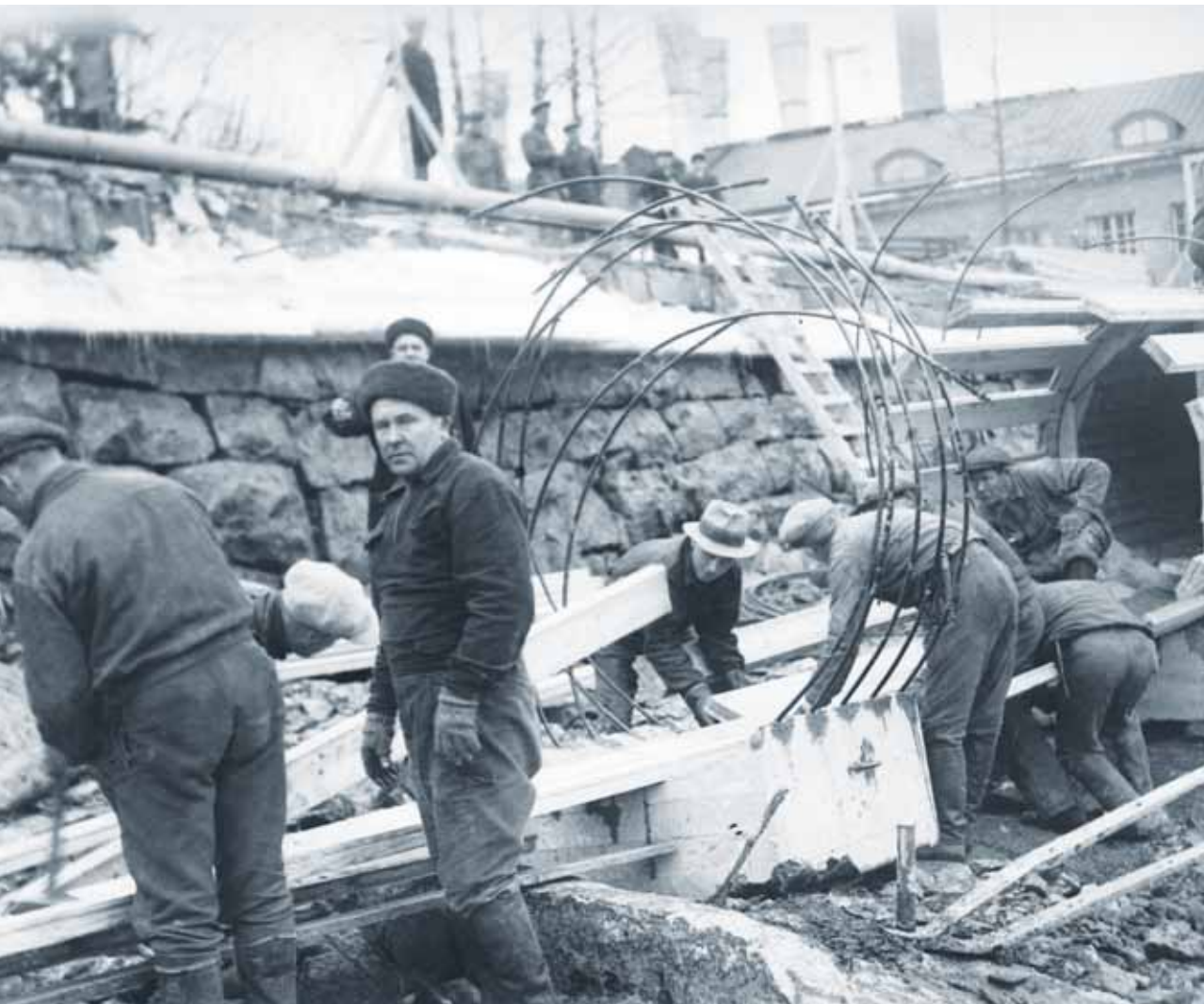
In the 1930s, Yleinen Insinööritoimisto built wooden water intake pipes for companies in the forest industry. These pipes provided factories with the utility water they required for their production processes from the closest lake or river.
