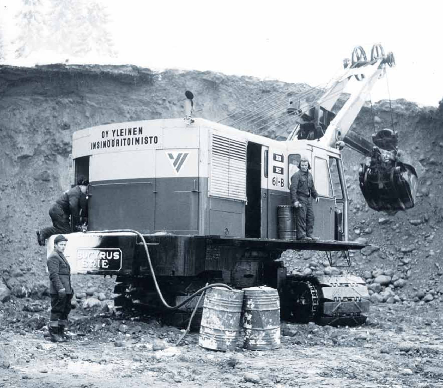
Yleinen Insinööritoimisto's Bucyrus Erie digger from the 1960s. Sand was required as a base material in highway construction.
