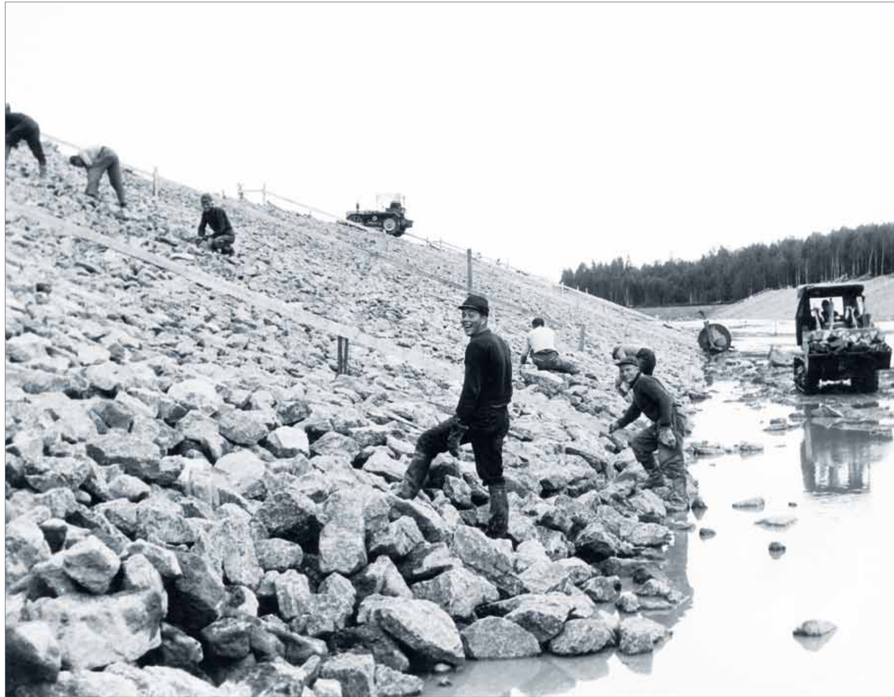
The Saimaa canal, which led from Finland to the Baltic Sea through the Soviet Union, was built in the 1960s. The stone banks of the canal were constructed using manual labour.
