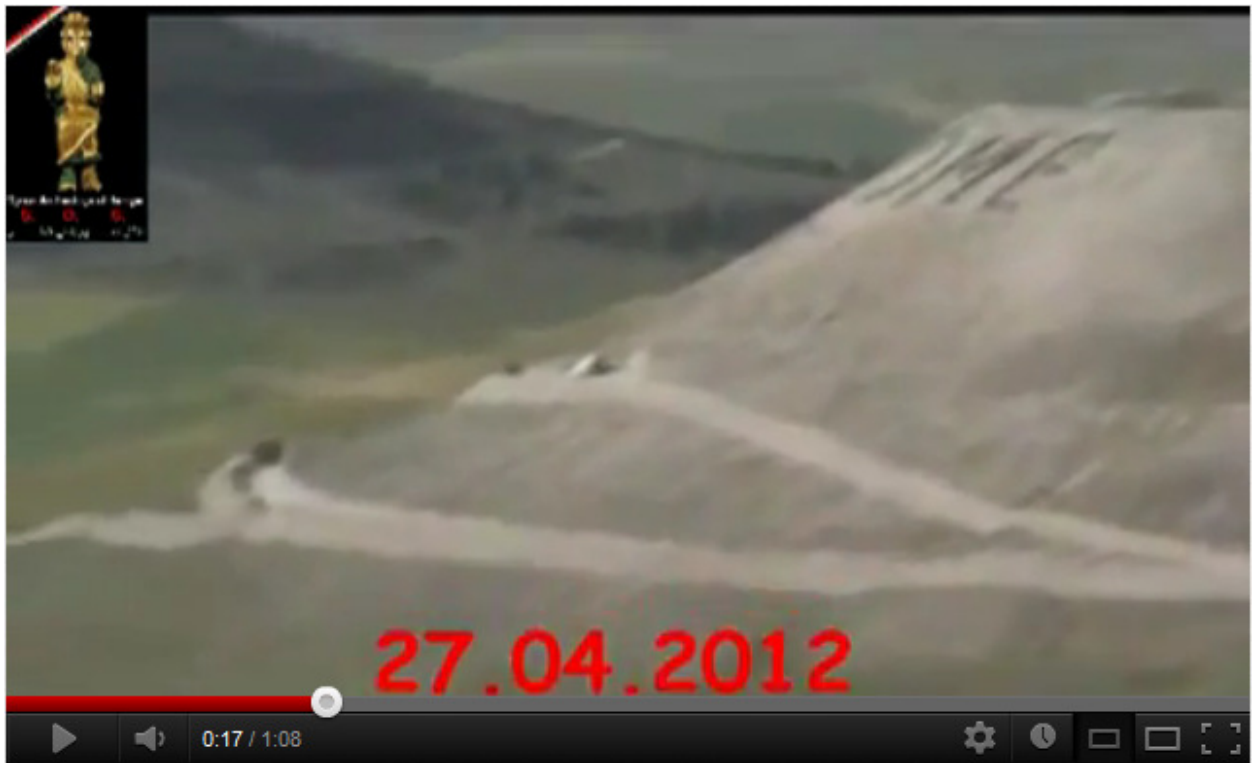
Figure 30: Embankments in the side of Shmemis Castle 209
