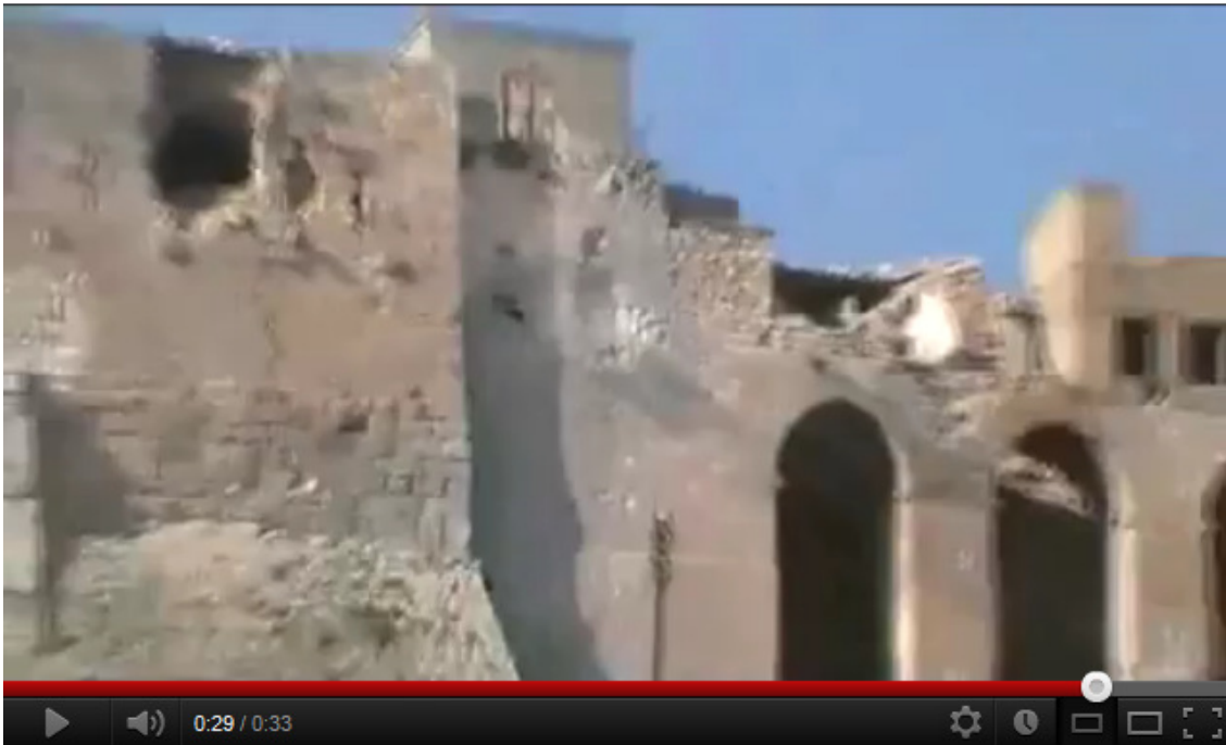
Figure 23: Damage to Qal'at al-Mudiq after prolonged shelling (26 March 2012) 146
