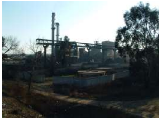
Iron and steel plant at Boksburg (4.1.6)
