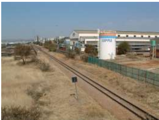
General view of industrial access line in
