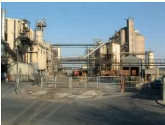
Food processing mill at Germiston South (4.1.14)
