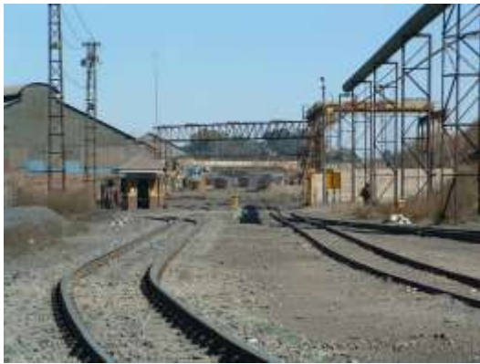
Iron and steel works railway lines, Powerville, Vereeniging (4.1.23)
