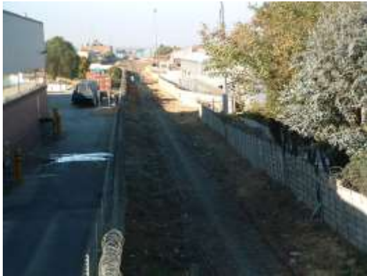
Alrode industrial area railway lines Being uplifted (4.1.1)
