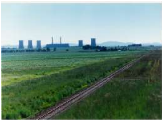
Grootvlei – Redan line, with Grootvlei Power station (3.2.6)
