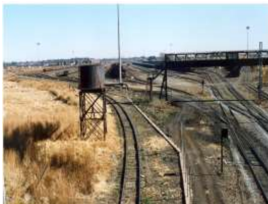
Steel facility receiving yard at Bijlkor, Vanderbijlpark. (4.2.27)
