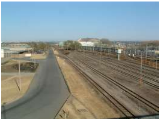
General view of access line and road at Boksburg East. (4.1.6)
