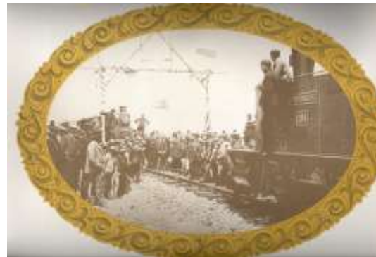
Opening of Durban - Johannesburg line near Heidelberg ( 3.1.6 )
