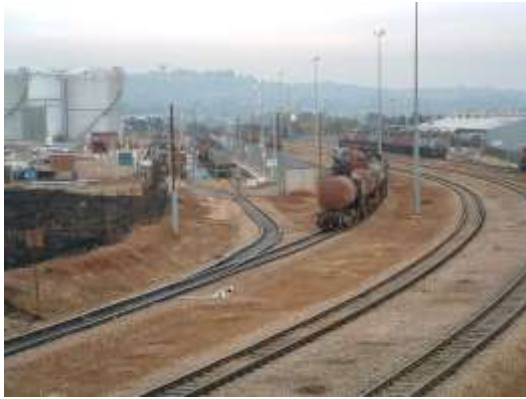
Multi-track yard at Waltloo fuel depot. (4.1.34)
