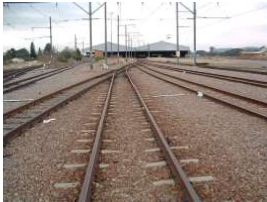
Disused former PX sheds at Capital Park, awaiting a new client. (7.3)
