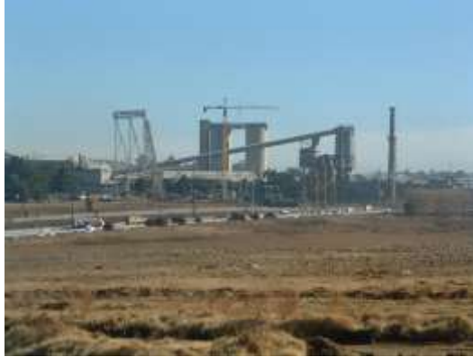
Jupiter cement works with N3 in foreground. (4.2.13, 3.1.8)
