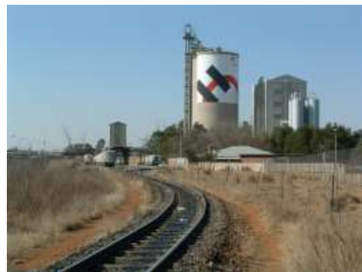
Bulk cement facility private siding, Vulkania, Brakpan. (4.1.32)
