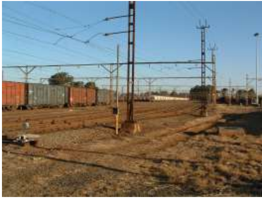
Natalsspruit yard with soda ash wagons for Alrode distributor ( Text ref: 4.1.1 )
