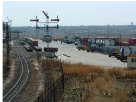
Eastcon container depot, Dunnotar. (3.2.1, 6.4)
