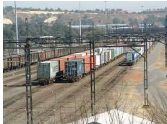
Kaserne yard with container trains. (7.7)
