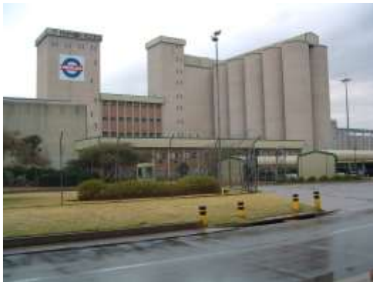
Waltloo Mill. Rail deliveries reduce road congestion in area. (Text reference: 4.1.34)
