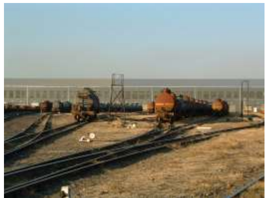
Germiston wagon repair depot. (9.3.2)
