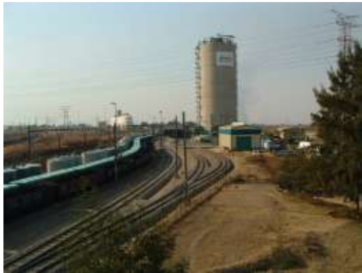
Wagons of bulk and palletised-bagged cement at large Kaalfontein distribution point. (Text reference: 4.2.14, 3.1.1)
