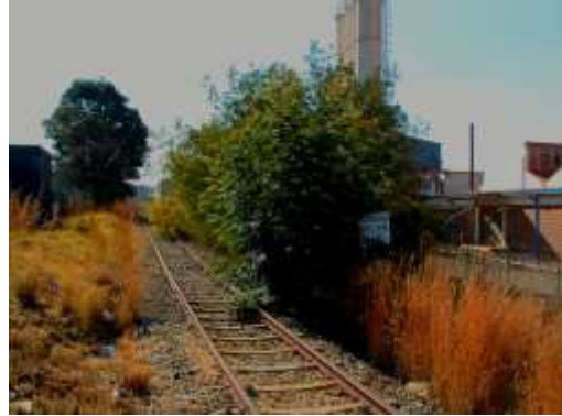
Access line overgrown and disused at Factoria, Luipaardsvlei. (4.1.13)
