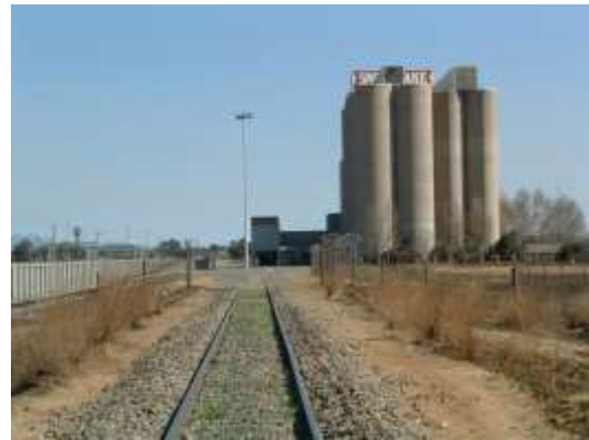
Mill and railway lines at Leeuhof, Vereeniging (4.2.16, 3.1.9)
