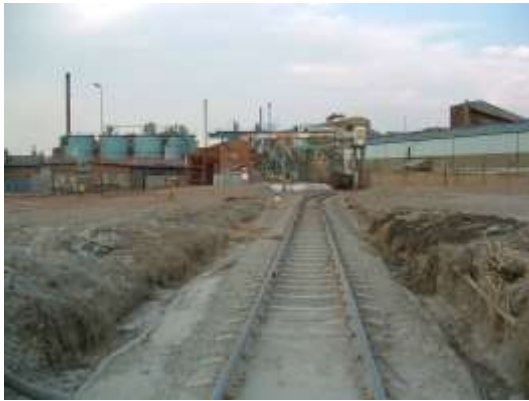
Zinc smelting works at Struisbult, south of Springs. (4.2.24, 3.2.1)
