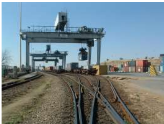
City Deep, portal gantries for loading or offloading between rail and road. (6.1)
