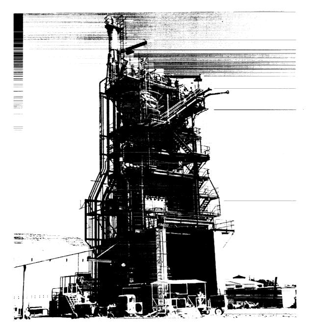
Figure 14. - M-1 Rocket Engine Project - Thrust Chamber and Gas-Generator Test Stand C-9.
