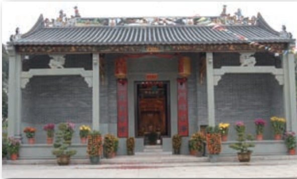
The two eave columns attached to the walls of the façade, Man Ancestral Hall, Tai Hang (Photography by Lo Wai Ling)
