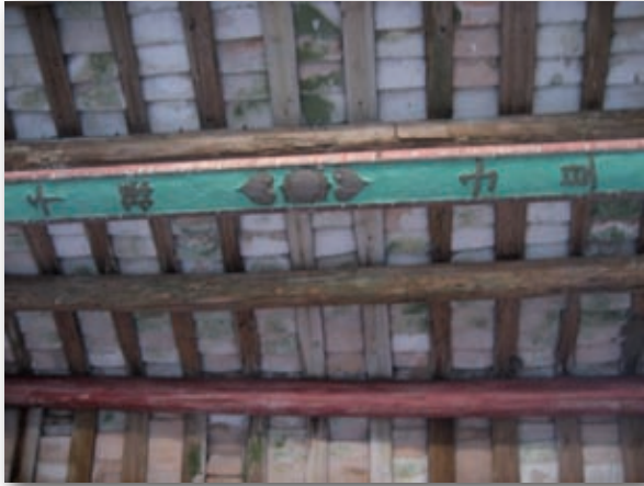
Lantern beam, Leung Ancestral Hall, Ma Po Mei Village (Photography by Tsui Yuen Ling)
