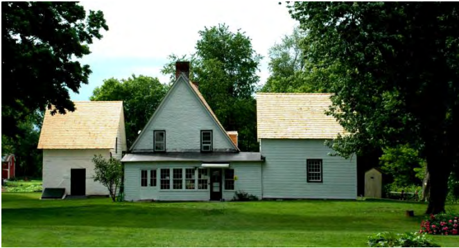
Mabee Farm buildings with their new cedar roofs
