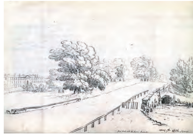
JC Nattes: bridge on Rotten Row 1801.
