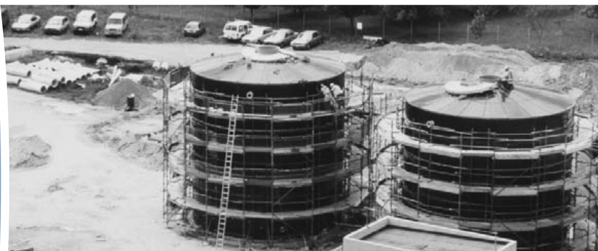
The new digester building under construction at the Wastewater Treatment Plant.
