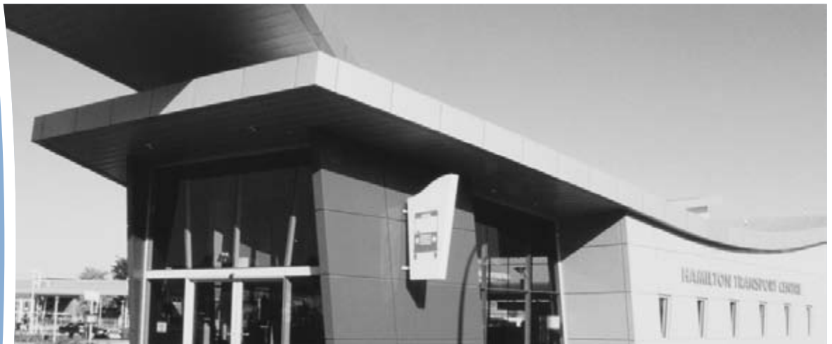
Hamilton's latest strategic facility-the Hamilton Transport Centre.
