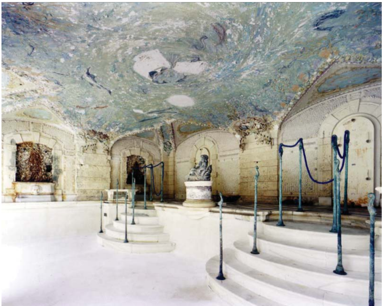
Figure 6.8. Ceiling above the swimming pool at Vizcaya (EverGreene, 2006).
