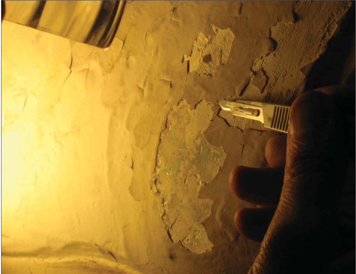
Figure 7.1. On-site paint exposure with a scalpel, conducted by Frank Matero (L. Drapala, 2009).
