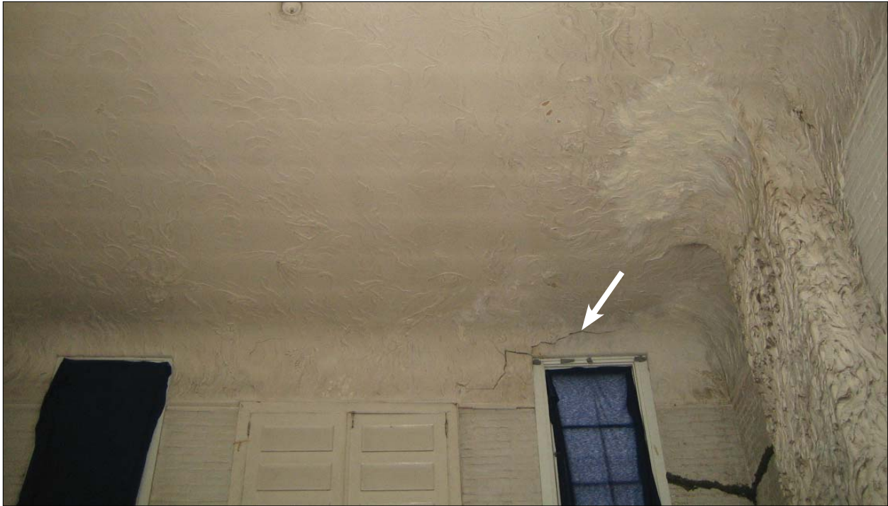
Figure 5.4. Ceiling cornice prior to cornice loss, November, 2006 (Archives of the New York Studio School).
