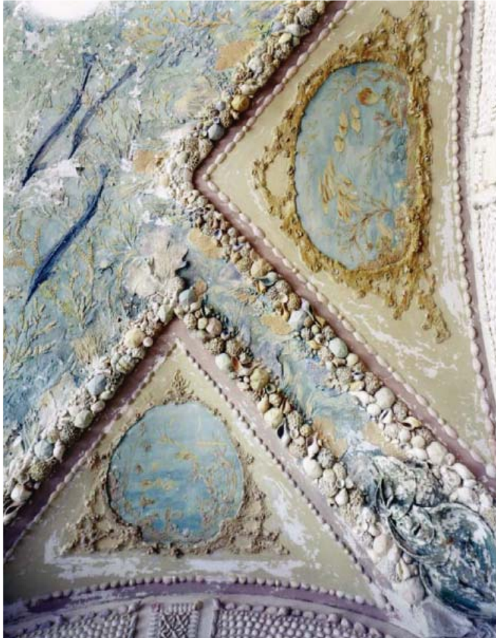
Figure 6.8. Detail of the high relief elements on the ceiling above the swimming pool at Vizcaya (EverGreene, 2006).
