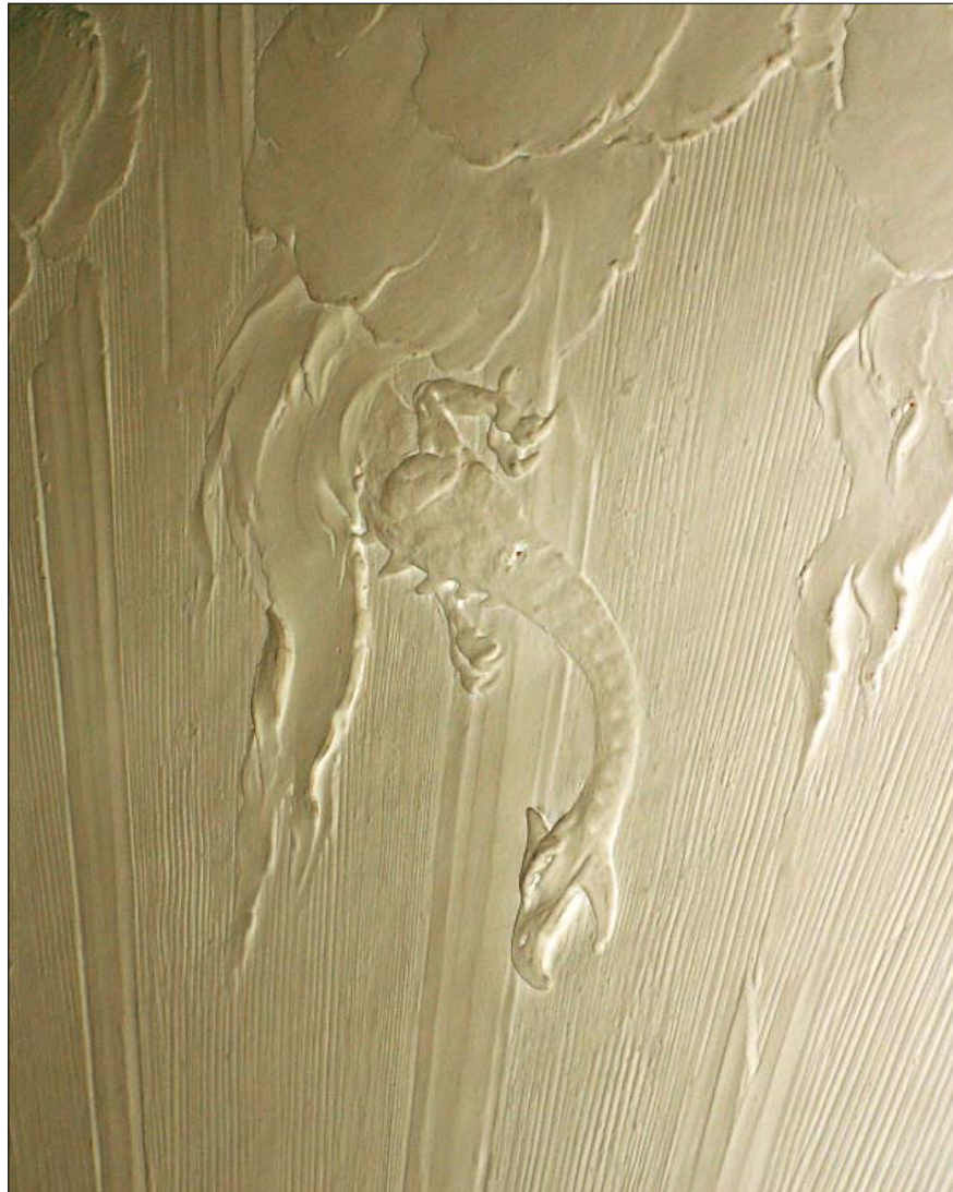
Figure 4.5. Griffin (relief appliqué) with exposed nail used to fix piece. The over tooled background surface (in situ applied rays and ridges) continues under the pre-cast figure, with hand-applied reliefwork (flames and clouds) used to conceal the edges of the appliqué (L. Drapala, 2009).
