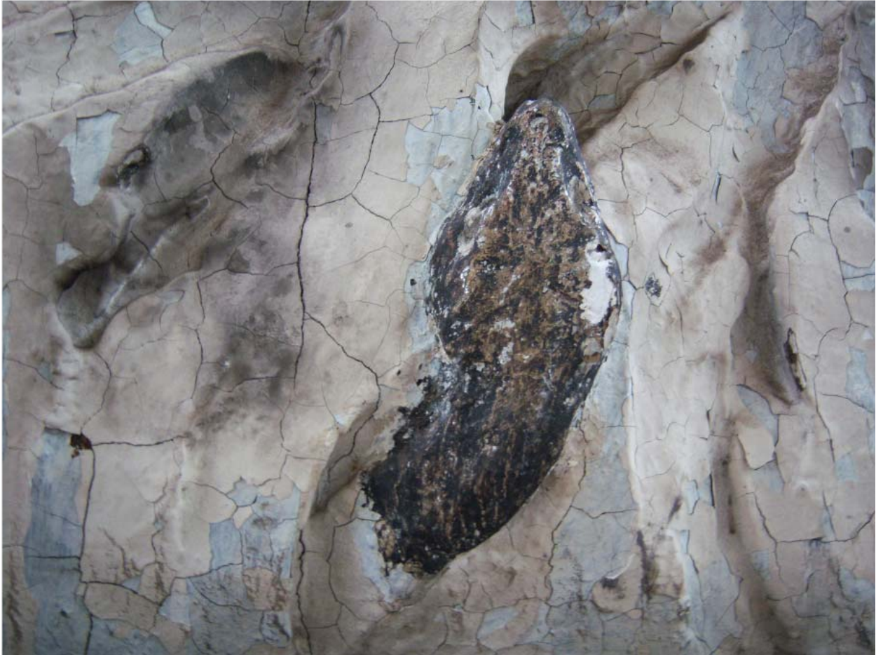
Figure 7.2. Exposure of a flame element on the fireplace, exposing black paint over a metallic finish. This was most likely uncovered during the 1999 Alan Farancz investigation (L. Drapala, 2009).
