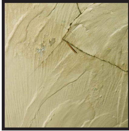
(a) crack monitoring
