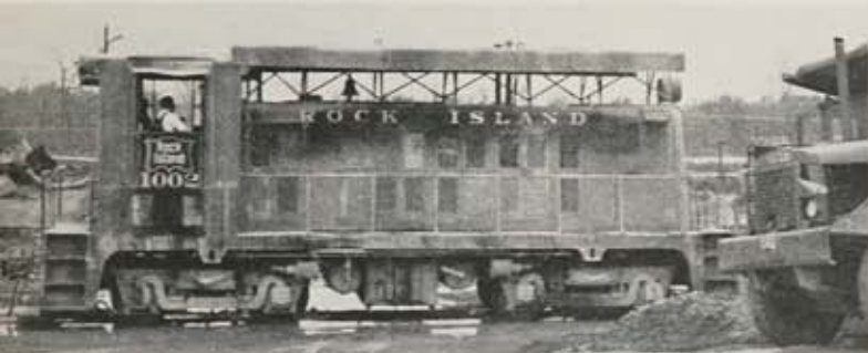
ONE of Rock Island's unique 1200 h.p. B-B EMD TA's speeds across Oklahoma with the Choctaw Rocket (above). Ex-Canadian National Whitcomb 1002 wears a protective shield while on lease to Big Rock Gravel at Little Rock. Firm later purchased the 75-ton Dominion diesel unit.
