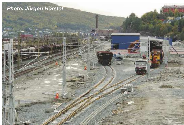
In January 2006 work started on a new ore discharge facility, SILA, at the site of the shunting yard for ore trains in the actual terminal. There are 11 underground silos for ore, and one for additives. They have a diameter of 40 m and a depth of 60 m, and the discharge hall is 600 m long, the track running on a bridge above the silos. Between 1.3 and 1.5 million tonnes of ore can be stored. Conveyors run from the silos to the screening plant and quays. The left-hand photo, taken on 1 September 2006, shows excavation in progress, while by 17 September 2009 (right) the work was nearing completion, with the excavations filled in and track laid through the unloading hall with hot-water shower for de-icing to facilitate unloading, on the right.
