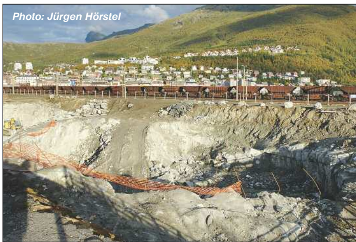
In January 2006 work started on a new ore discharge facility, SILA, at the site of the shunting yard for ore trains in the actual terminal. There are 11 underground silos for ore, and one for additives. They have a diameter of 40 m and a depth of 60 m, and the discharge hall is 600 m long, the track running on a bridge above the silos. Between 1.3 and 1.5 million tonnes of ore can be stored. Conveyors run from the silos to the screening plant and quays. The left-hand photo, taken on 1 September 2006, shows excavation in progress, while by 17 September 2009 (right) the work was nearing completion, with the excavations filled in and track laid through the unloading hall with hot-water shower for de-icing to facilitate unloading, on the right.
