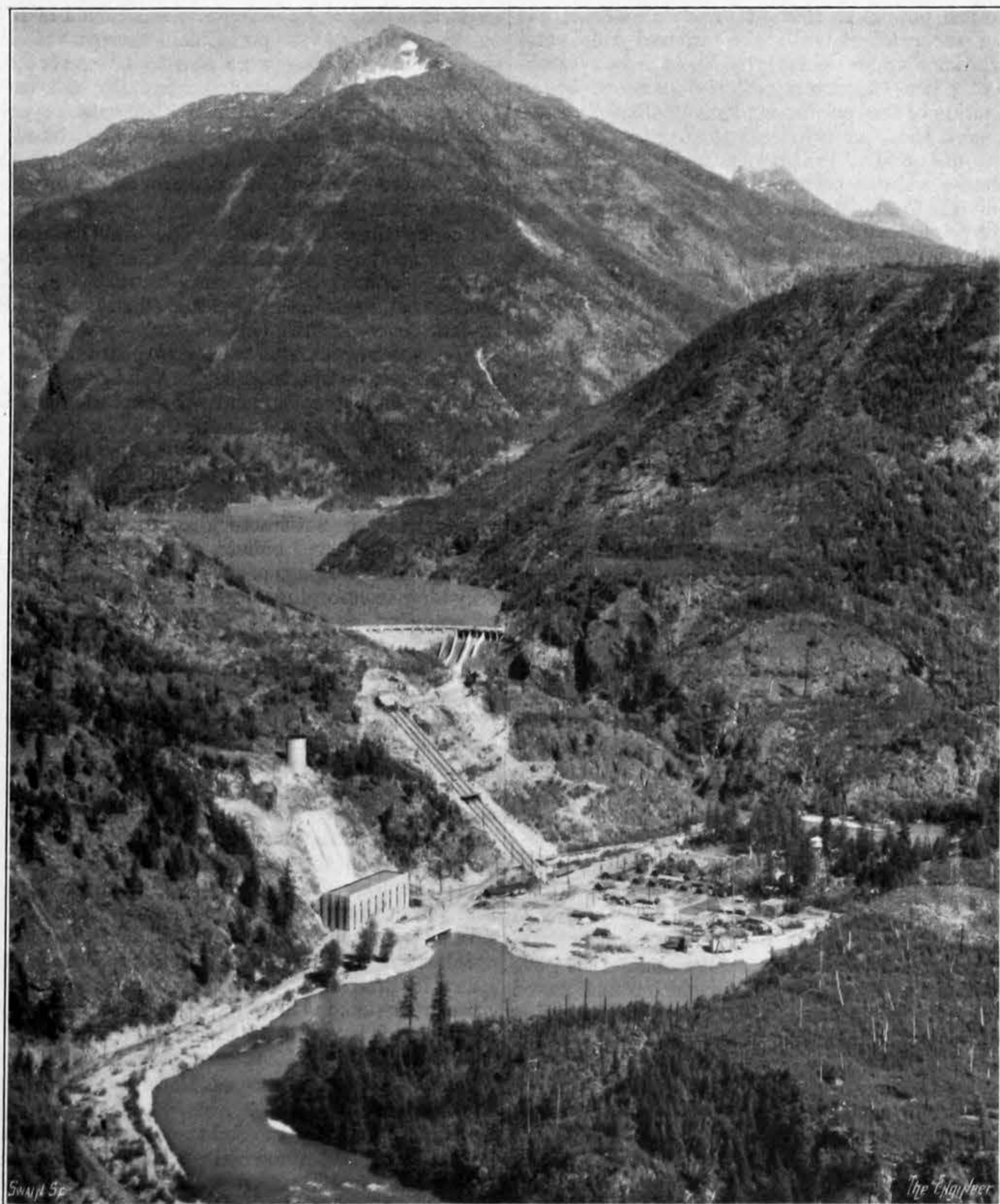
FIG. 4—DIABLO DAM AND POWER-HOUSE
