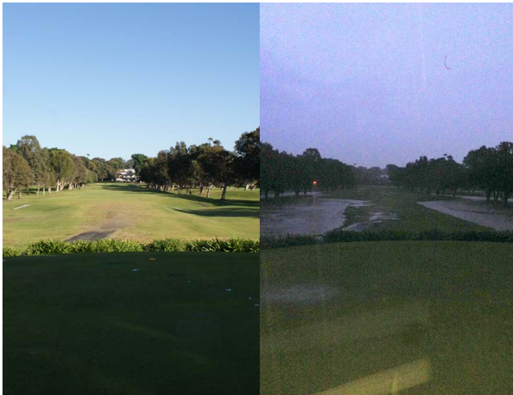
Detention basins in good weather & retention basins in flooding
