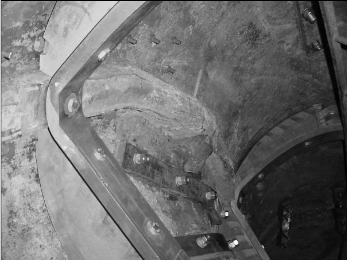
Fig. 2 New bronze reinforcements within the left arm of the Bavaria statue.
