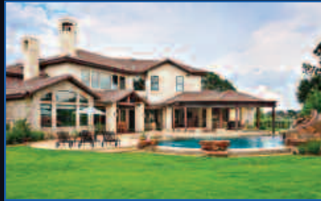
Custom Home Outdoor Living Space MORNING STAR BUILDERS
