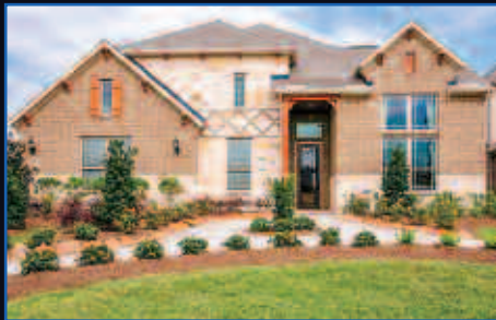
Volume Builder Product Design $300,000 to $350,000 GEHAN HOMES FINALISTS: Ashton Woods Ashton Woods
