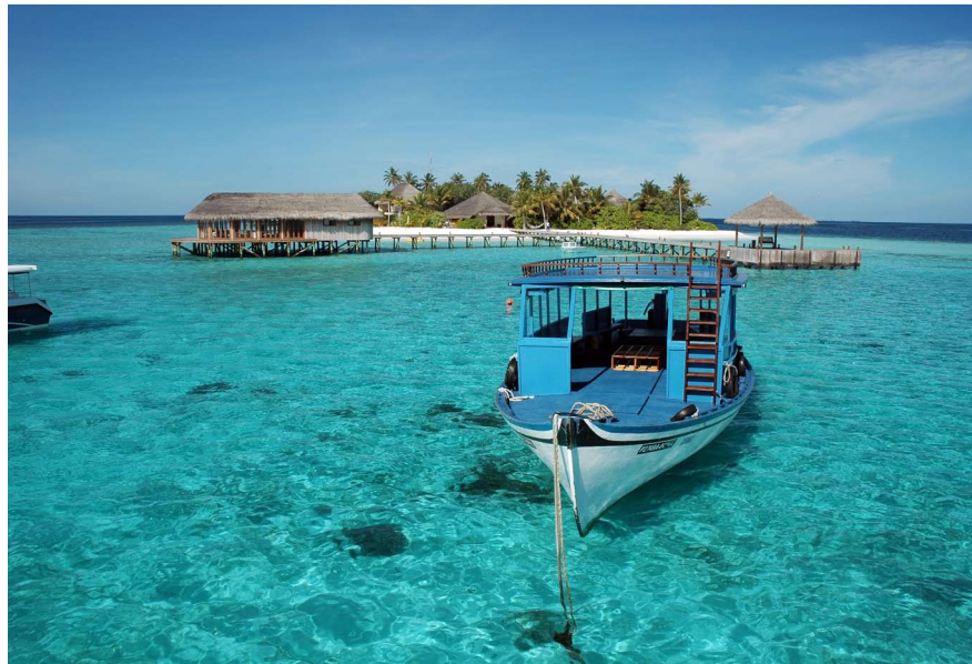
All major infrastructure in resort islands are generally in close proximity to coastline due to their small size.
