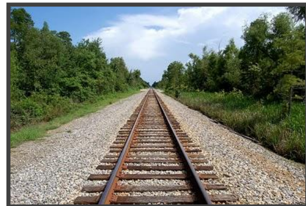
The gauge is the distance between the rails on a railroad. The U.S. Standard Gauge is 4'8 1/2"
