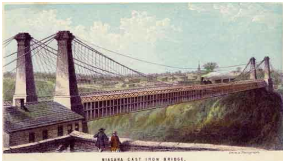
The Niagara Falls Suspension Bridge provided direct access to the state of New York and featured two decks, an impressive feat at the
