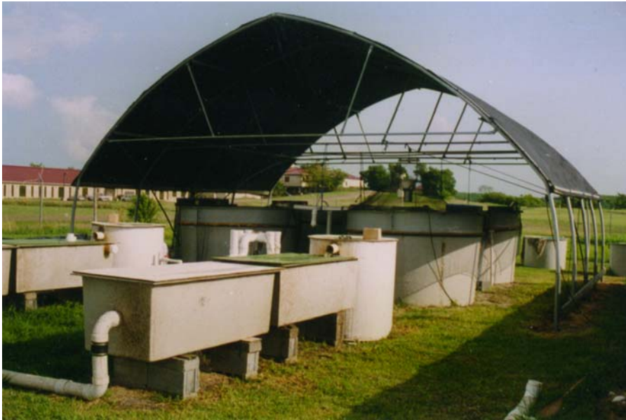
Fish rearing tanks, clarifiers and biofiltration tanks (in front of photo) at the UVI Agriculture Experiment Station
