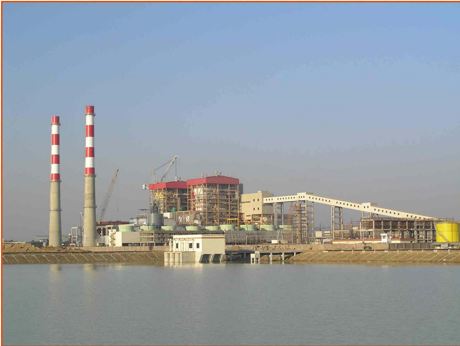
Barapukuria 2x125 MW Coal fired Power Plant
