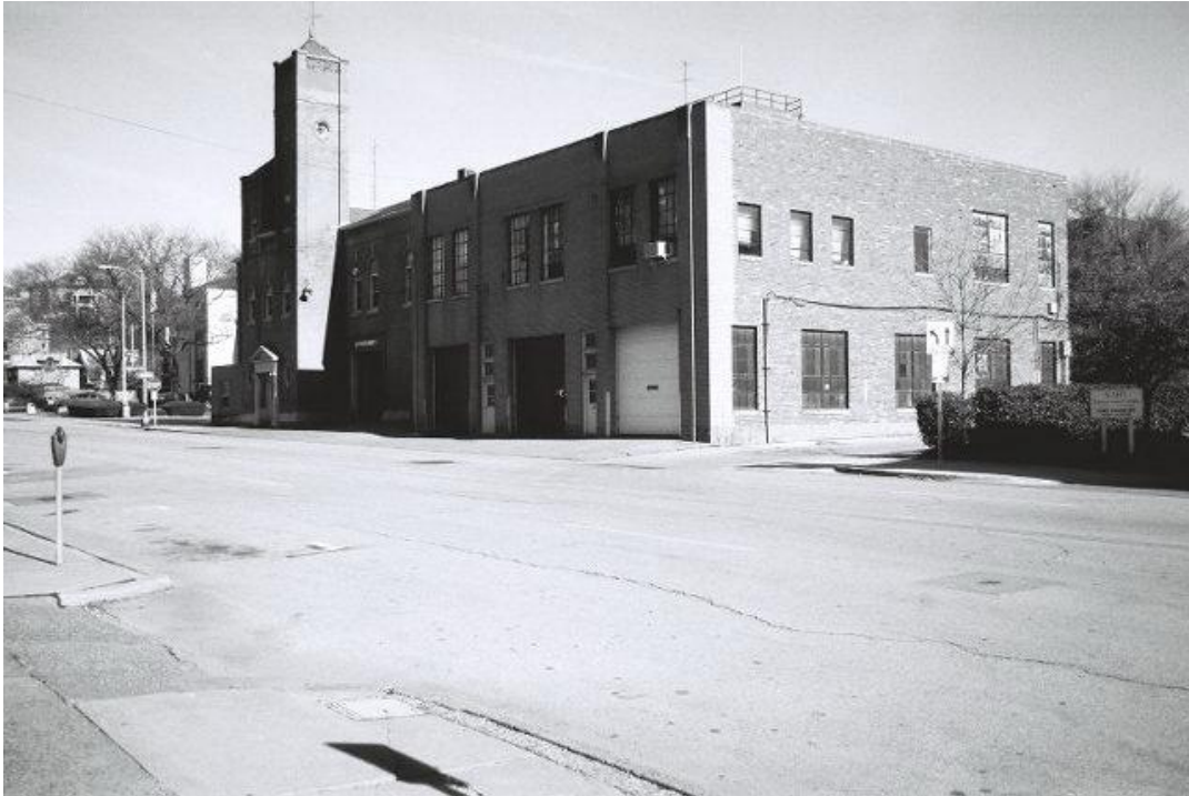
View of the west and south elevations, looking northeast across Scott Street. From this perspective, the three-bay addition to the rear is evident.
