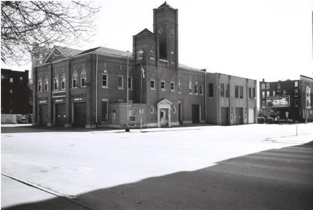
View of the north and west elevations, looking southeast across the intersection of West Fourth and Scott Streets.
