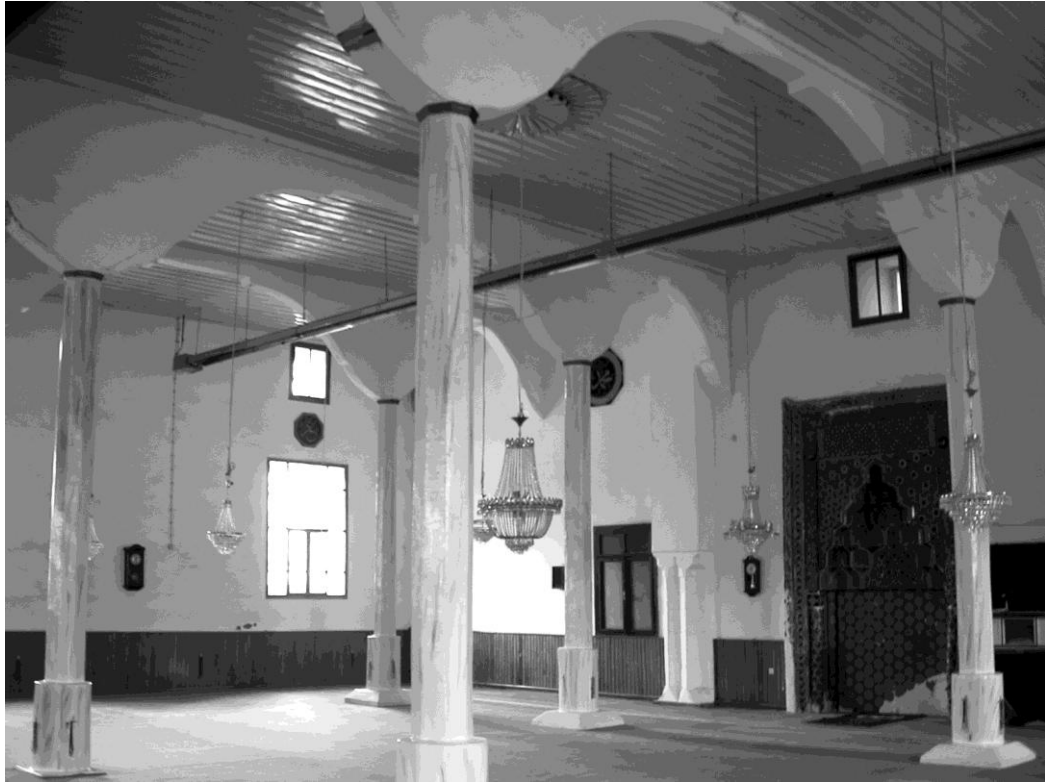
Fig. 15. Interior of the Sahip Ata Cami as reconstructed in AD 1871 by Muheddin Usta (now demolished). The mihrap is original, and the window between the mosque and the Sahip Ata's tomb can be seen east of the mihrap.
