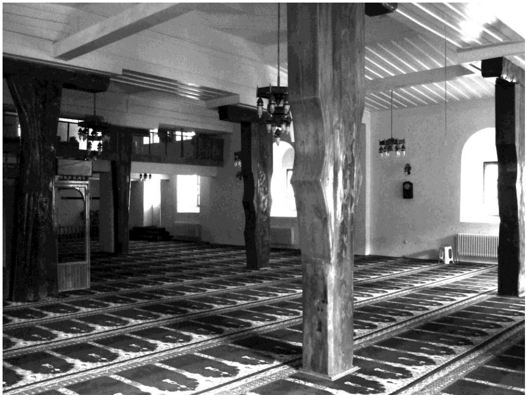
Fig. 10 The Tuğrul Şah Cami, İspir. Interior with four wooden columns and 'bindirme' roof. The column in the background was added when the north wall was removed.
