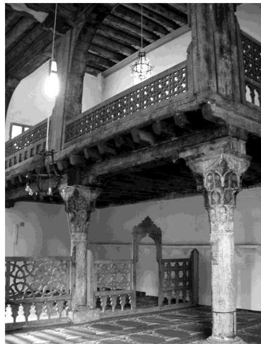
Fig. 48. The Emir Mahfil. Note that the volume breaks through the roof plane, which makes it legible from the exterior. The raff is on the side wall, behind the screen; the çilehane is located under the floor beneath the mahfil. The emir's door is out of the picture to the right, at the base of the stairs.
