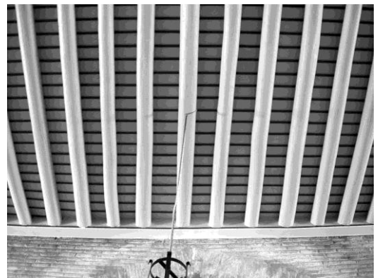
Figure 12 Wooden roof structures in Anatolian mosques. Top: Interior space and roof joists of the Ulu Cami, Sivas; Bottom: Interior space and roof joists of the Aladdin Cami, Konya. Note that in both cases the buildings are heavily restored and none of the wooden elements are original; it is unclear if the spacing, scale and (lack of) ornamentation accurately reproduces the original.
