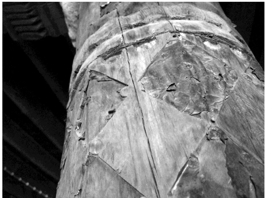
Fig. 32 Applied sheet metal ornament, Sivrihisar Ulu Cami.
