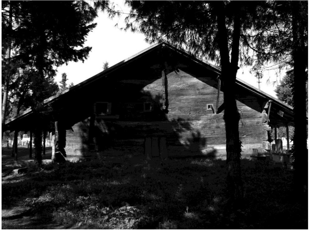
Fig. 07 Gökceli Cami, Çarşamba. Exterior view of kibla wall, showing quoin corners and the gable brace piercing through the pediment.
