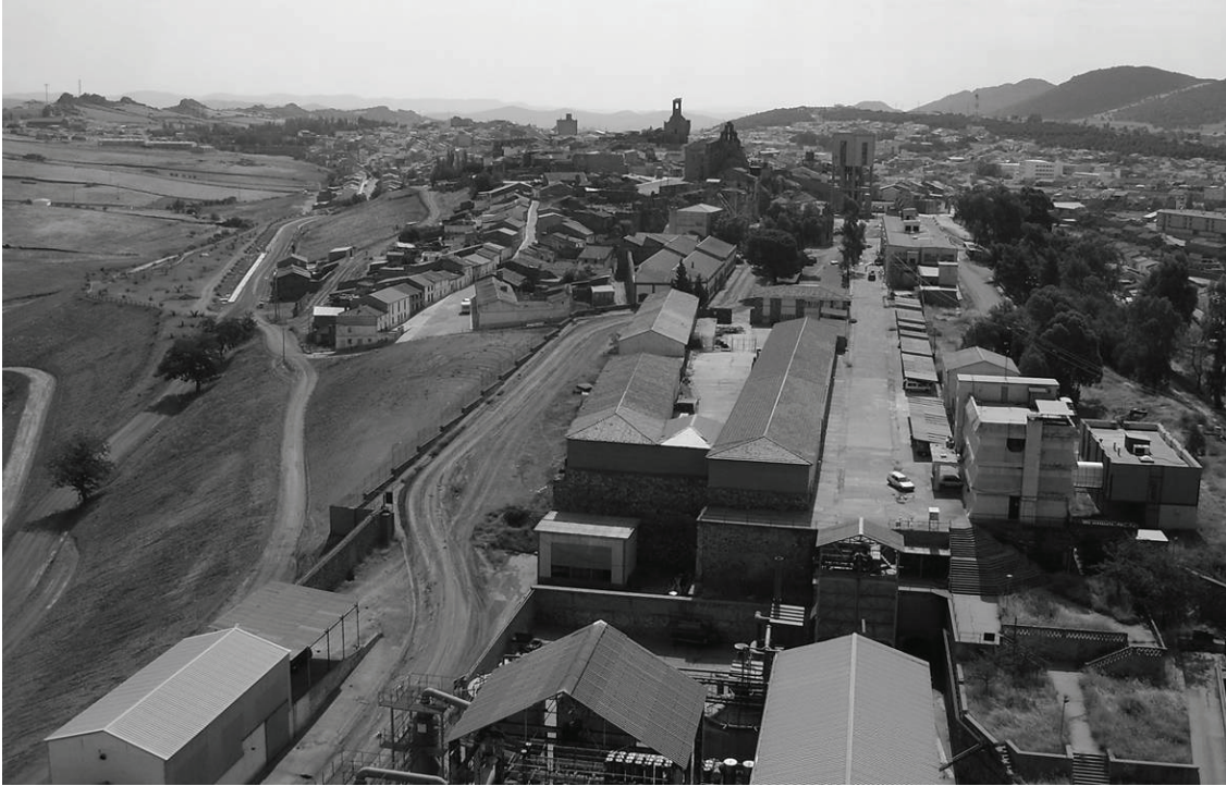
Almadén and the mine - Spain
