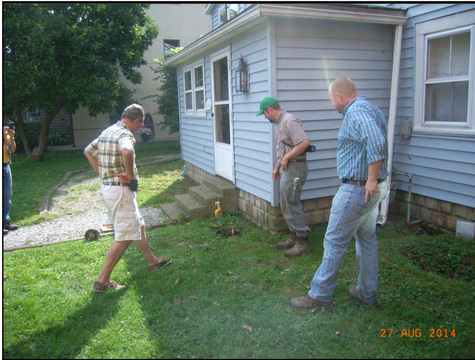
BUCKEYE LAKE 25 AUGUST 2014 Photo 045 – Residence at Station 112+25 with several depressions at the ground surface possibly from boils. Soil was very soft and groundwater was very shallow at this location.
