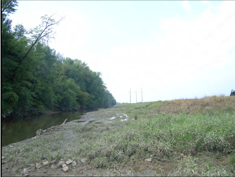
BUCKEYE LAKE 25 AUGUST 2014 Photo 043 – South Fork Licking River channel (facing upstream) after ODNR widening project. Note the recent deposition. A maintenance program will be essential to maintain conveyance capacity.
