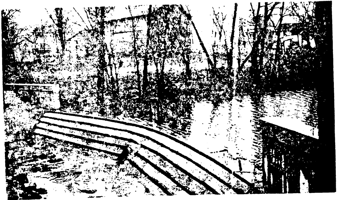
View of stilling basin dam located in outlet canal below spillway
