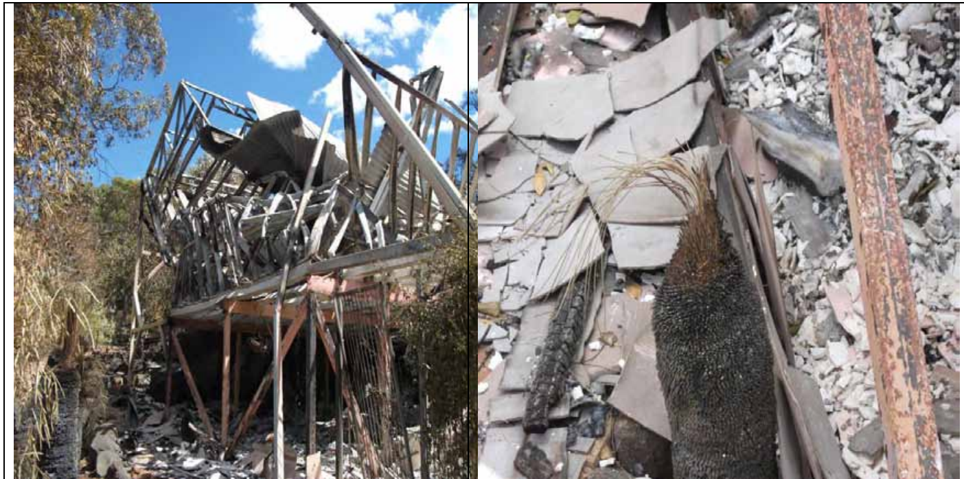
Figure 27: House constructed with cellulose cement cladding
