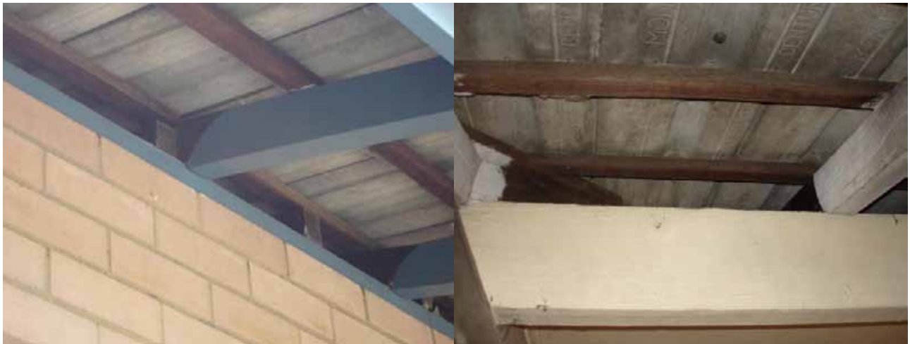
Figure 17: Further examples of the openings between the roof and the ceiling
