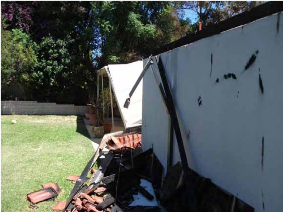
Figure 23: The BPZ closer to the house and the house featured in photograph 19.
