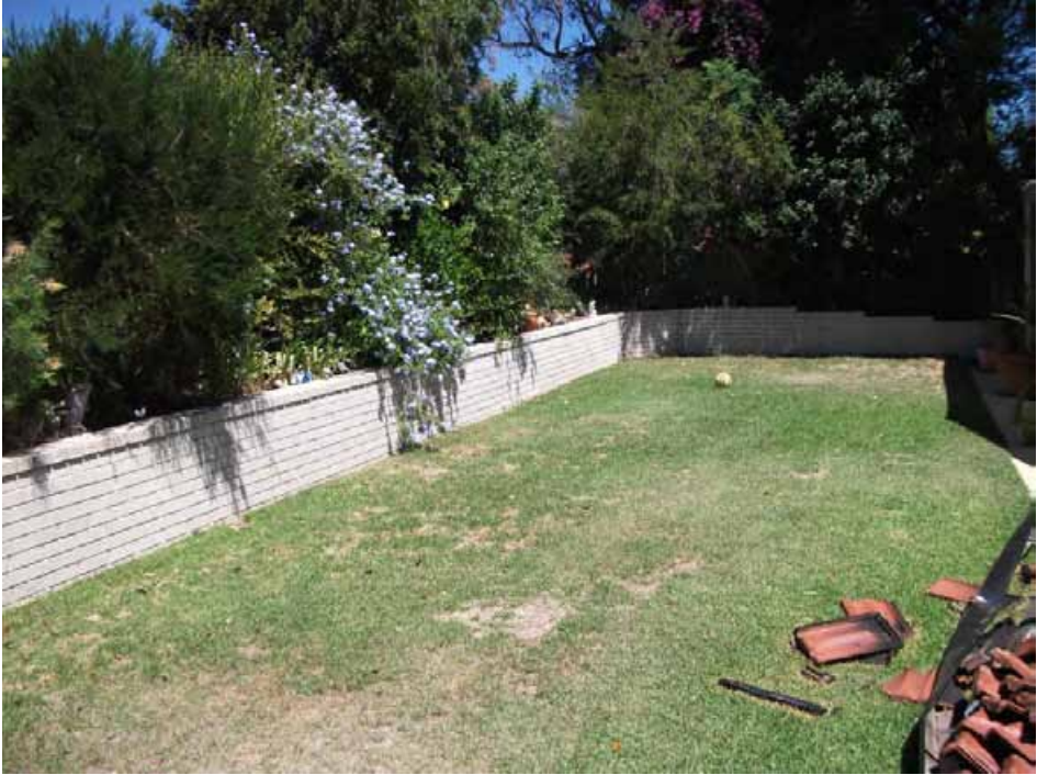
Figure 22: The building protection zone (BPZ) of a home destroyed as consequence of the ember attack
