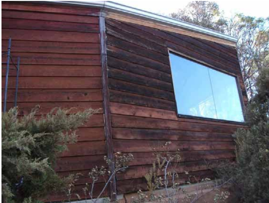
Figure 21: The cedar timber shed on similar construction style and materials adjacent to the destroyed cedar timber home.
