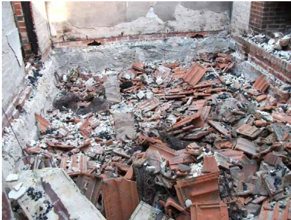
Figure 15: This is indicative of the flooring structure where the floor was wooden and supported around 30-45 cm off the ground
