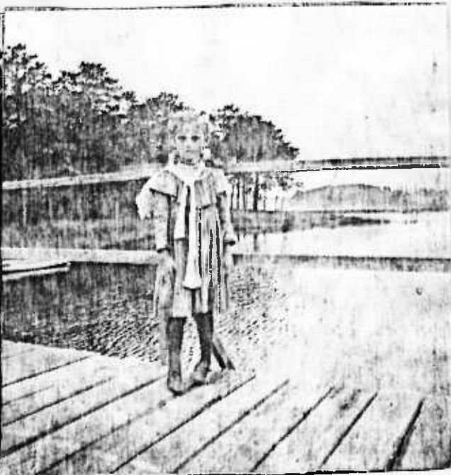
Bridge looking east
