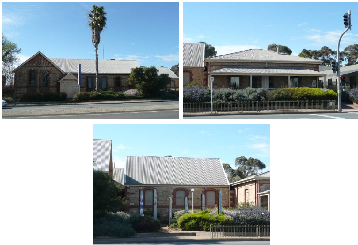
Views of former school buildings from Main North Road
