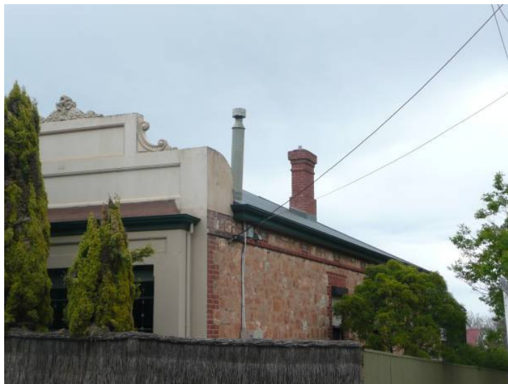
View of detail of front parapet to shop
