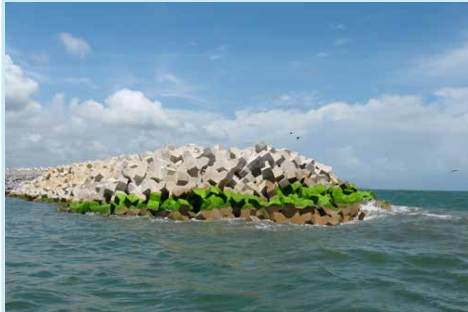
Figure 8-1: Typical design breakwater head
