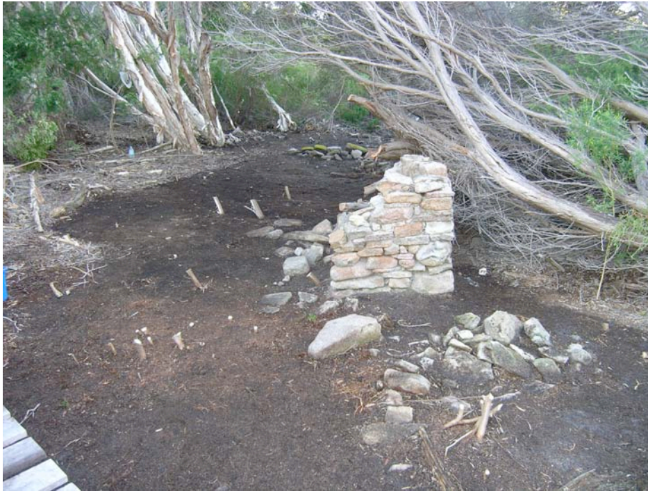
Figure 8. Clearing the site of vegetation: after. (Paterson 2006)
