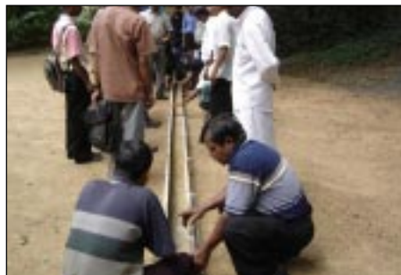
A training program on concrete pole manufacturing for micro hydro societies in September 2005 in Sri Lanka
