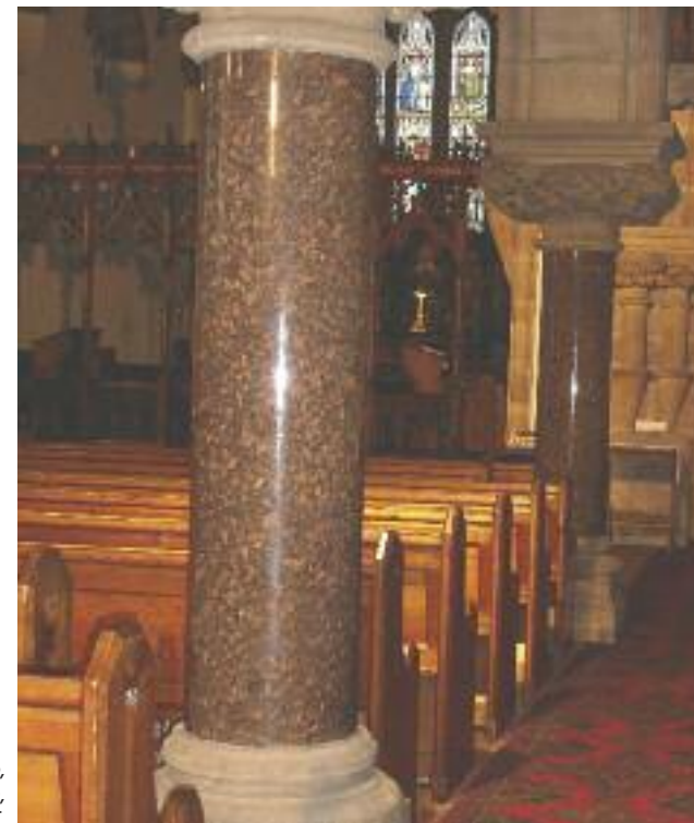
Pillars of polished Shap Granite, St Augustine's Parish Church, Alston. © B. Young, BGS, NERC.
