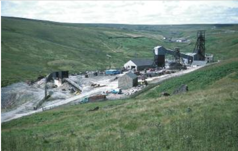
"Surface plant, Groverake Mine (now disused), Rookhope" © B. Young, BGS, NERC.
