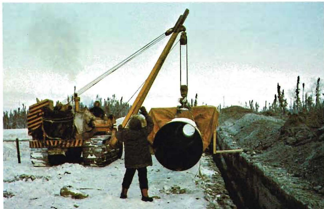
Forty-eight-inch-diameter pipe is lowered into place at test site.
