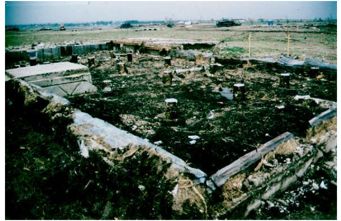
Home cleaned from pier and beam foundation
