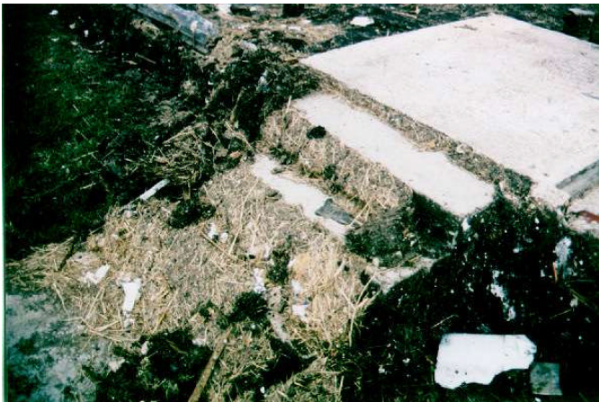
Grass "packing" turned front stairs into a ramp
