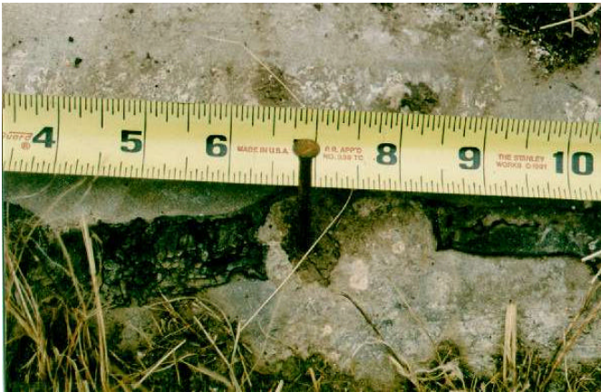
Concrete nail which secured bottom plate to slab
