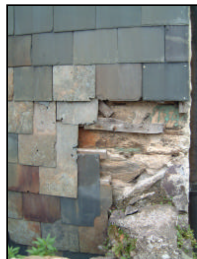
Top: an example of the use of local stone cobbles in paving. Above: a typical Georgian frontage in Bridge Street. Below: damage to a slate-hung wall. Finding suitable replacement materials
