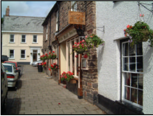
There is a mix of building materials and methods throughout the conservation area. Left : local stone is either left exposed or rendered using smooth (background) or roughcast render (foreground). Right : roofs are mainly of Welsh slate or varieties of clay pantile (e.g. double-Roman tiles), some replacing earlier thatch. Slate has in turn sometimes been re-
