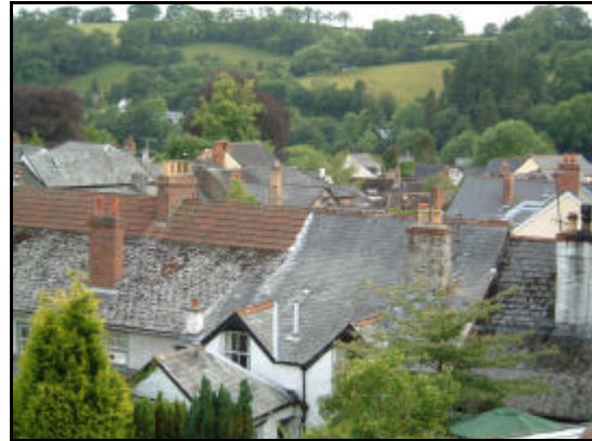
There is a mix of building materials and methods throughout the conservation area. Left : local stone is either left exposed or rendered using smooth (background) or roughcast render (foreground). Right : roofs are mainly of Welsh slate or varieties of clay pantile (e.g. double-Roman tiles), some replacing earlier thatch. Slate has in turn sometimes been re-
