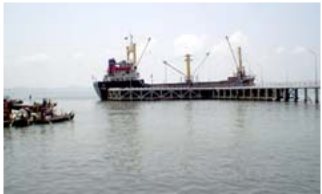
Sittwe Harbor—Main Wharf
