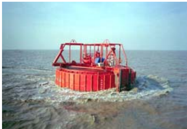
Hazira Offshore Terminal SPM
