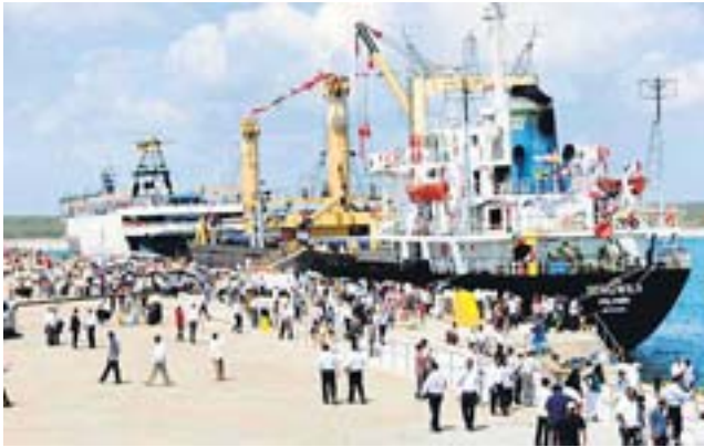
Magampura Port—General Cargo Quay
