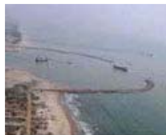
Karaikal Port Breakwaters
