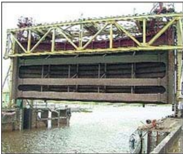
Lock Gate at Bhavnagar Port
