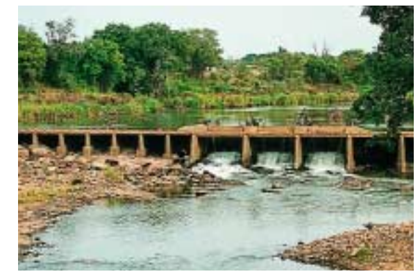
Large weirs disrupt flows in river systems: apart from impeding fish migration, they cause bank scouring, sedimentation and loss of riparian vegetation.
