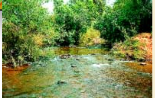
A large new weir is under construction at Xikundu as part of the Nandoni Scheme. A fishway has been incorporated into the design of the weir, motivated by the high diversity of rare and sensitive species found in this area.
