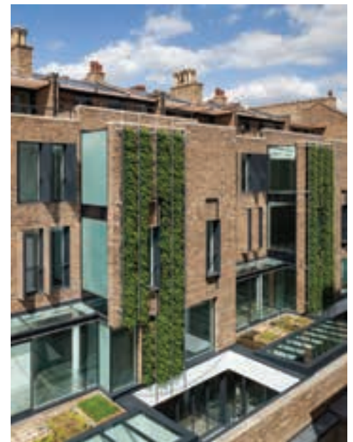
20 BENTINCK STREET – GREEN WALL
