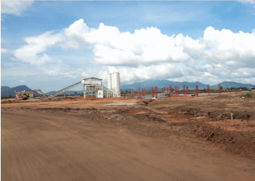
Project construction near Ngapidat village
