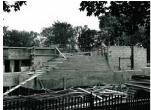
Construction of CNA House
