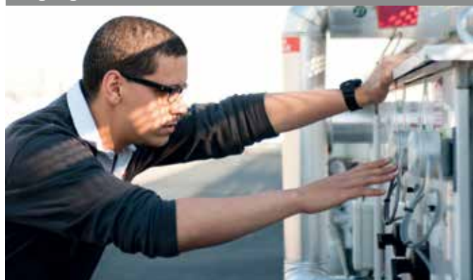
Ongoing checks at our data centres
