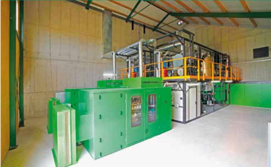
URBAS-Holzgas-KWK-Anlage HVG V12A 150 GLS URBAS HVG V12A 150 GLS wood gas CHP plant
