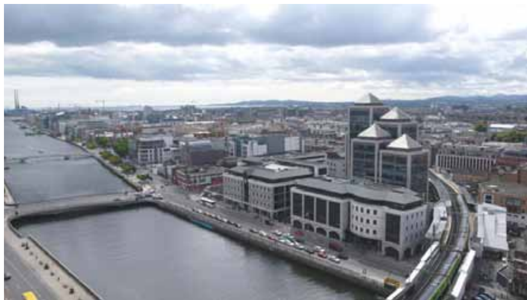
Figure 3.17 George's Quay and Tara Street Station /Loophline Bridge
