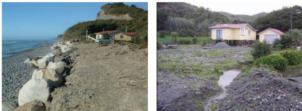
Figure 6.7: Relocation of a property back from the eroding coastline on the West Coast.
