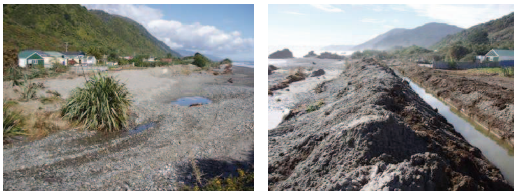
Figure 3.2: Wash-out of the gravel barrier on the west coast of the South Island during a storm in 2006 has significantly increased the risk of inundation due to wave run-up and overtopping to the properties that back the beach.
