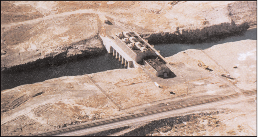
West Desert pumping plant. Water was pumped from the north arm of the lake through a 4.1-mile-long canal to the 320,000-acre West Pond.
