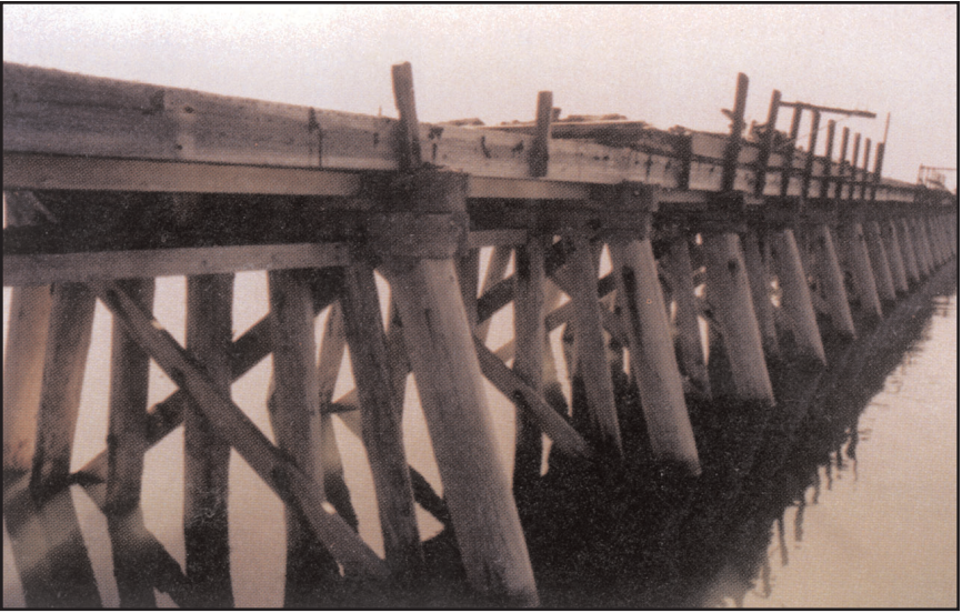
Original wooden trestle railroad that crossed Great Salt Lake, constructed about 1903. Photo by June Cannon, Cannon Structures, Inc.. A salvage operation for the wood started in 1993; some is used in the lobby of the Department of Natural Resources.
