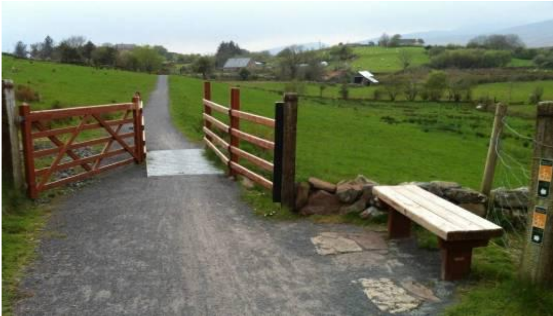
Example of the Great Western Greenway in Mayo, un-fenced across a sheep grazing field, and with animal grid at the entry point.
