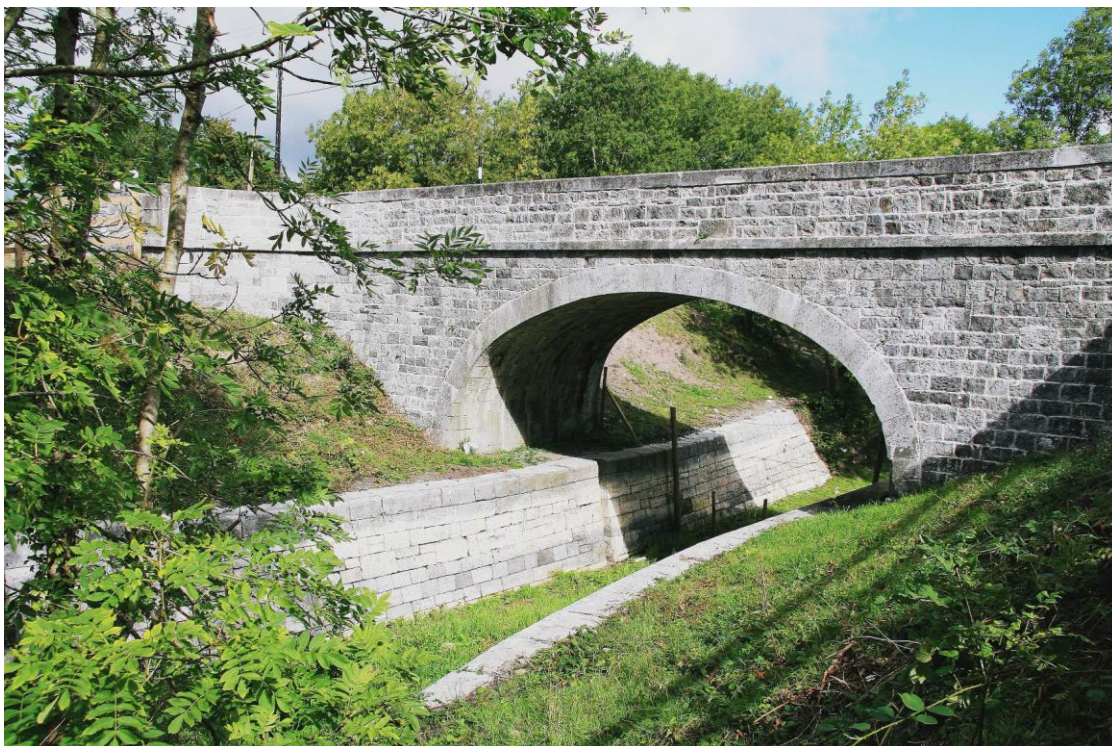
Figure 2.3 Poolboy Bridge over the disused Grand Canal
